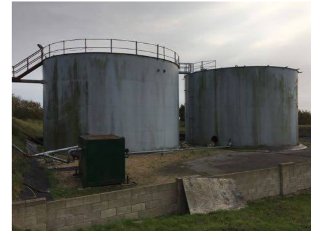
Photo 12. Buildings B67 and B68
