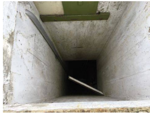
Photo 2. View into underground section of Building B1
