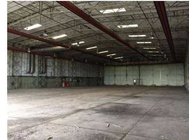
Photo 12. Interior of Building B11
