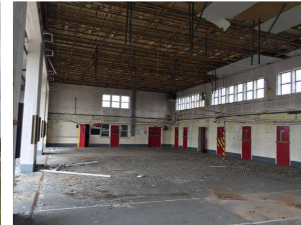
Photo 12. Interior of Building B52
