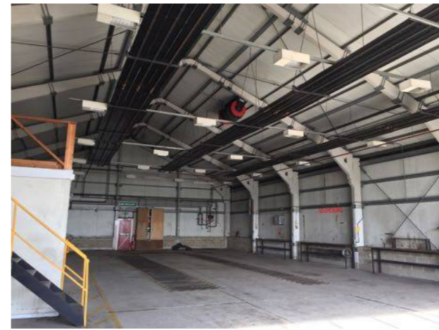
Photo 4. Interior of Building B17
