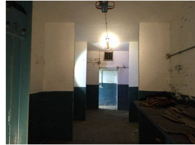
Photo 8. Interior of Building B8
