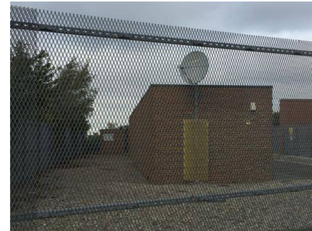
Photo 10. Buildings B37 and B38
