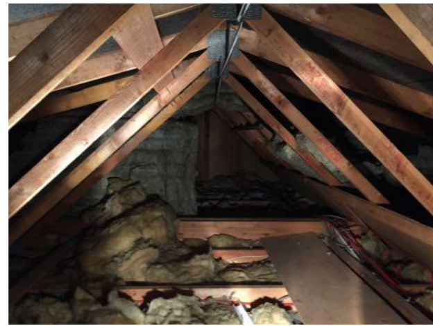
Photo 2. Roof void of Building B16
