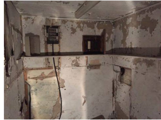
Photo 6. Interior of Building B33
