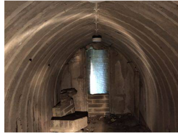
Photo 6. Interior of Building B18
