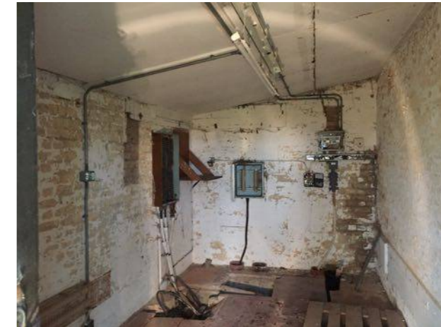
Photo 12. Interior of Building B39
