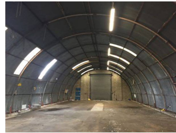
Photo 4. Interior of Building B45
